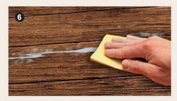
It is recommended to roughen the surface if over coating is required. Clean all equipments immediately after used with Kossan epoxy thinner 6.03.
