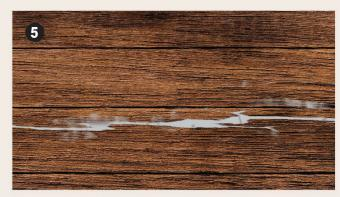
Remove the paper tape along the both sides immediately after the gap is filled.
