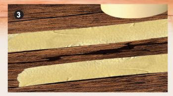
Use paper tape along the both sides of the gaps to obtain good strength filling.
