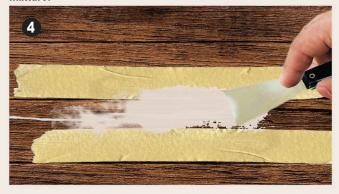
It is recommended to fill the gaps properly by squeeze the filler into the gap till it is full and remove excessive filler by scraper.
